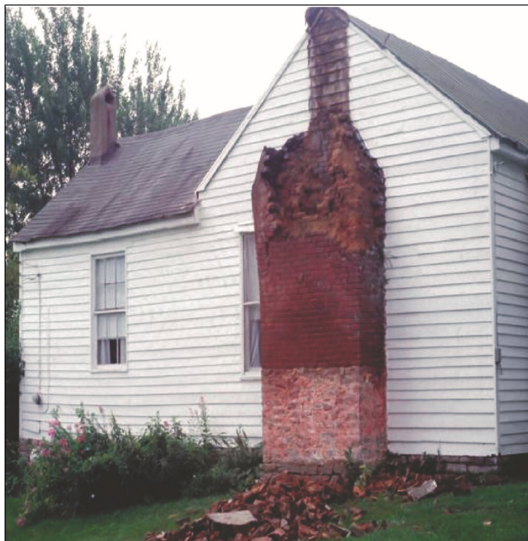
Figure 1-6. Chimney damage in Bath County caused by the ground motion (shaking) from the 1980 Sharpsburg earthquake.
